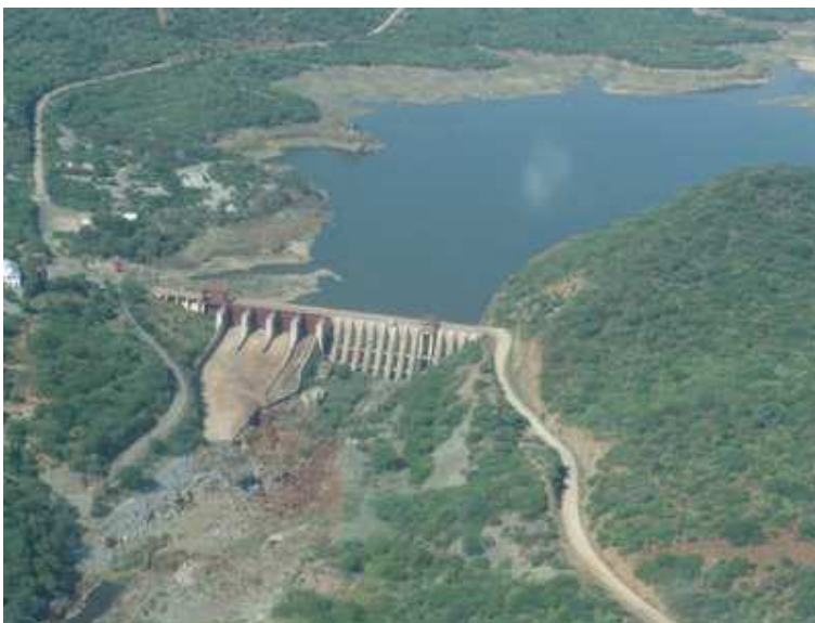
Fig. 2: Mtera dam in central Tanzania, the biggest hydroelectric facility of the country
